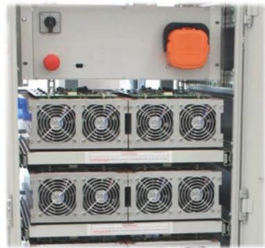
29) Full-custom high-performance battery cabinet (480 V, 320 A, 20 kWh, 100 kW continuous charge and discharge) based on lithium-titanate (LTO) prismatic battery cells able to operate at temperatures between -30°C and 55°C.
