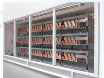
5) Modular multi-level converter with 66 sub-modules for static var compensation (SVC) in a medium voltage power grid (Source: Siemens)
