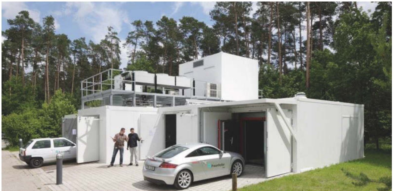
Fraunhofer IISB's electric vehicle test center
