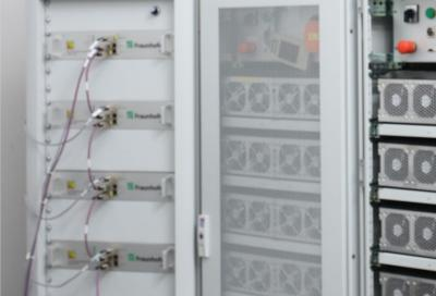
systems. The converters were deployed to interconnect a battery storage unit and a wood-working tool machine. Besides providing resiliency, the deployment of the active controlled storage system contributed to improve the total energy efficiency of the machine by up to 10 % by regenerative braking energy that would otherwise be dissipated into heat.
