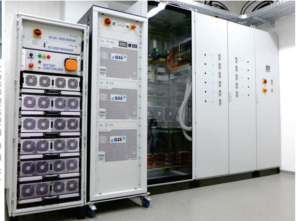
battery capacity: 3 racks with each 20 kWh AC/DC bridge with up to 100 kW HPDC-Distribution up to 1600 A / 800 V DC (on main bus bar)
