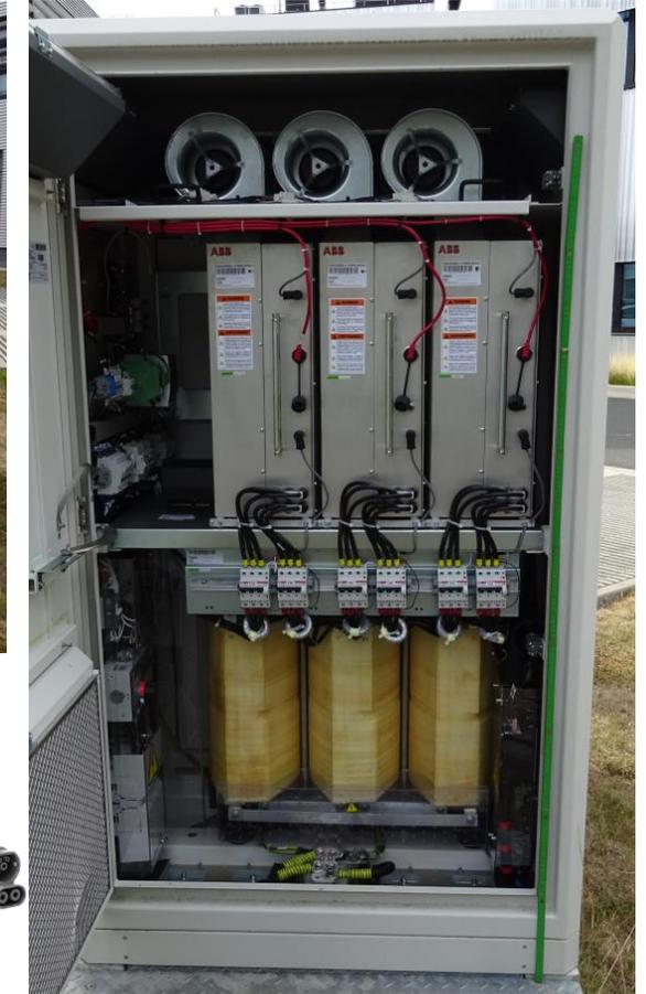
DCI4Charge specify DC Charging from a 650V DC-Microgrid
