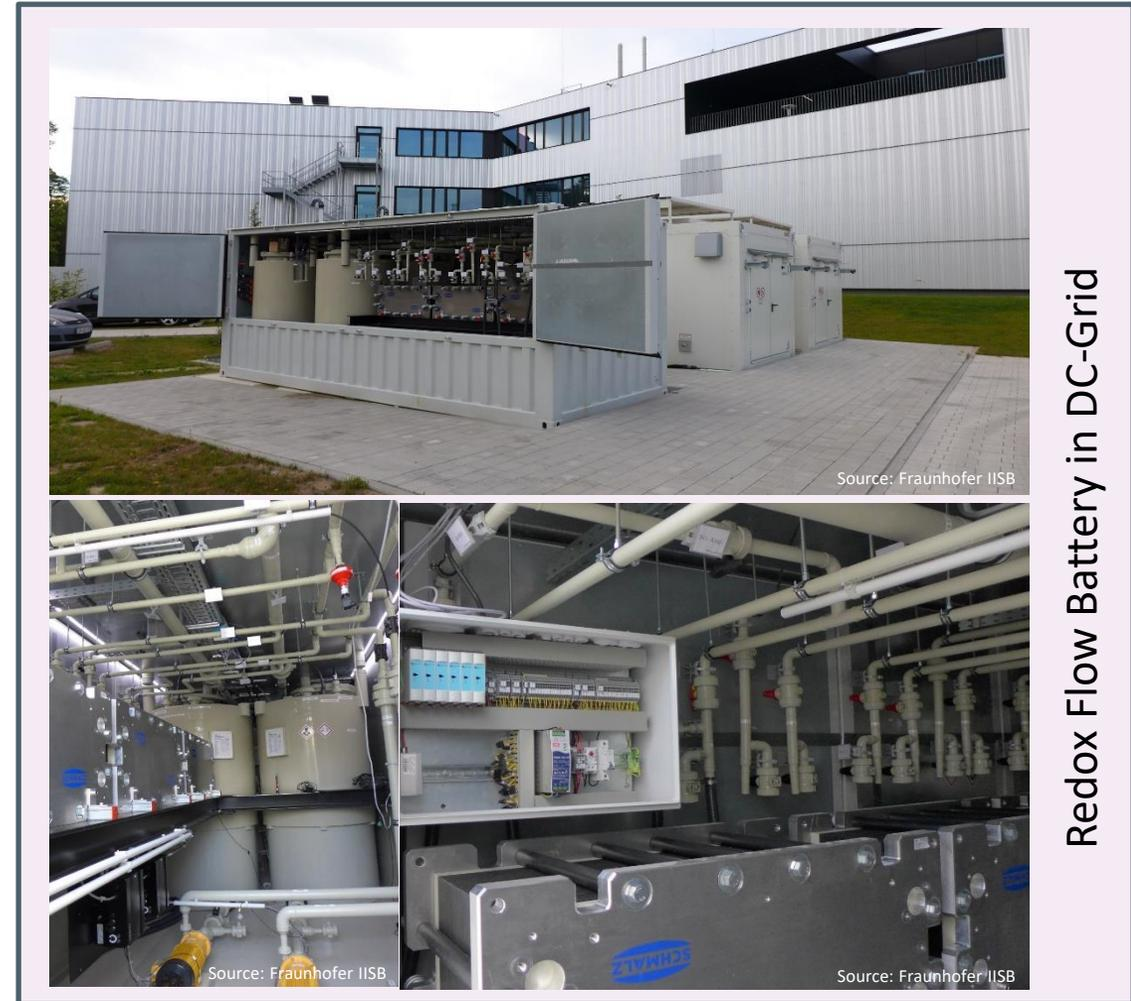
Redox Flow Battery in DC-Grid
