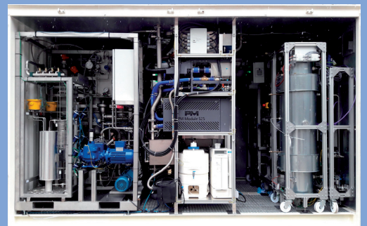
View inside the 20 ft container with electrolyser (left), fuel cell (center) and oneReactor (right)
